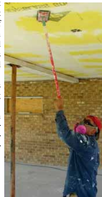
Mike Castaneda sanding drywall
